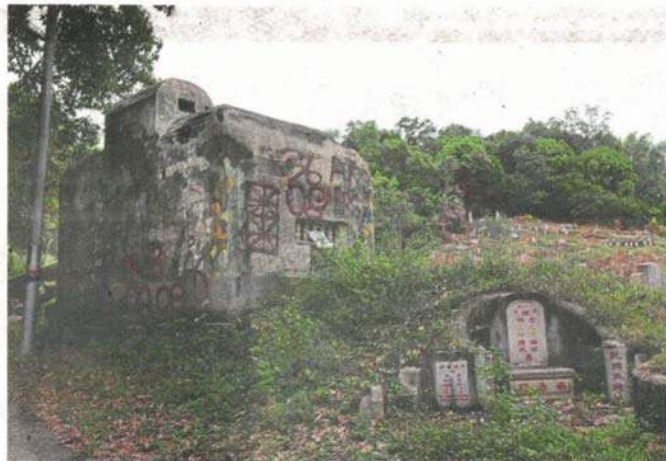
The pillbox at Mount Erskine cemetery has been vandalised.
